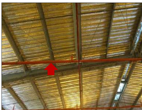
Water Deluge System / Water Spray System
